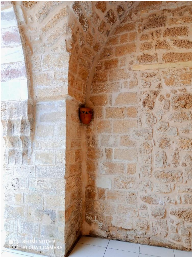
Fig. 10. Al-Ashi house, stone walls after removing cement plaster. (Source: Iwan Centre, 2021)
