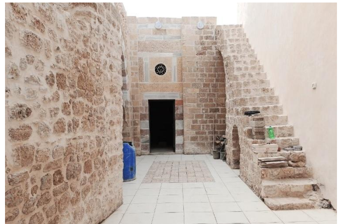
Fig. 12. Al-Ashi house, the courtyard after treatment. (Source: Iwan Centre, 2021)
