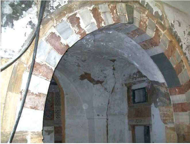
Fig. 9. Al-Ashi house, the arch of the iwan before restoration. (Source: Iwan Centre, 2011)
