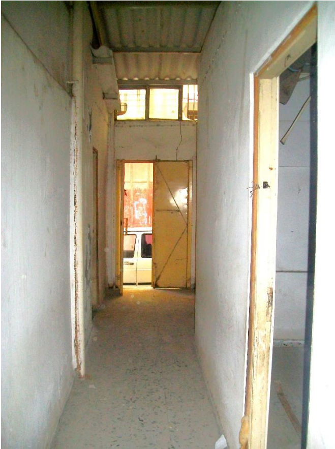
Fig. 8. Al-Ashi house, concrete blocks addition and the corridor. (Source: Iwan Centre, 2011)
