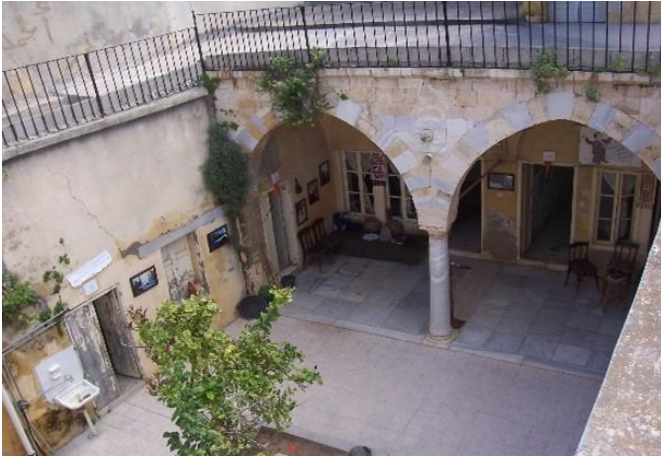
Fig. 1. Al Galayeni courtyard house with a riwaq, GOT. (Source: IWAN Centre, 2010)
