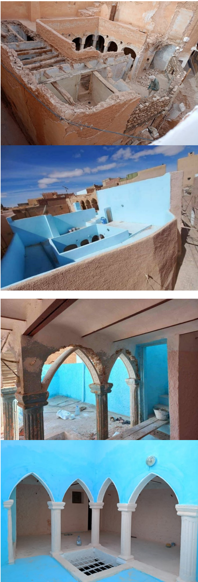
Fig. 5 (left). The rehabilitation operations for the historic ksour of the M'Zab Valley. From top to bottom: A) A dwelling before rehabilitation; B) the result of rehabilitation; C) a patio of a dwelling before the rehabilitation; and D) the result after rehabilitation. (Photos: The housing directorate of the wilaya of Ghardaïa, 2023)
