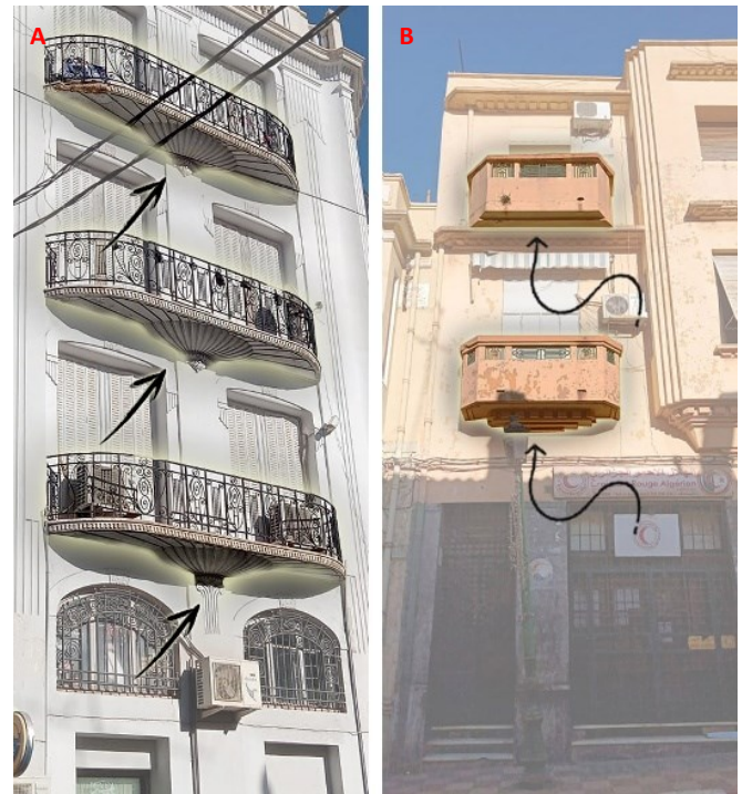
Fig. 12. Examples of an A2a typology balcony platform. A) A corbeil balcony; B) A balcony stoup with a dentile. (Source: Authors, 2024)
