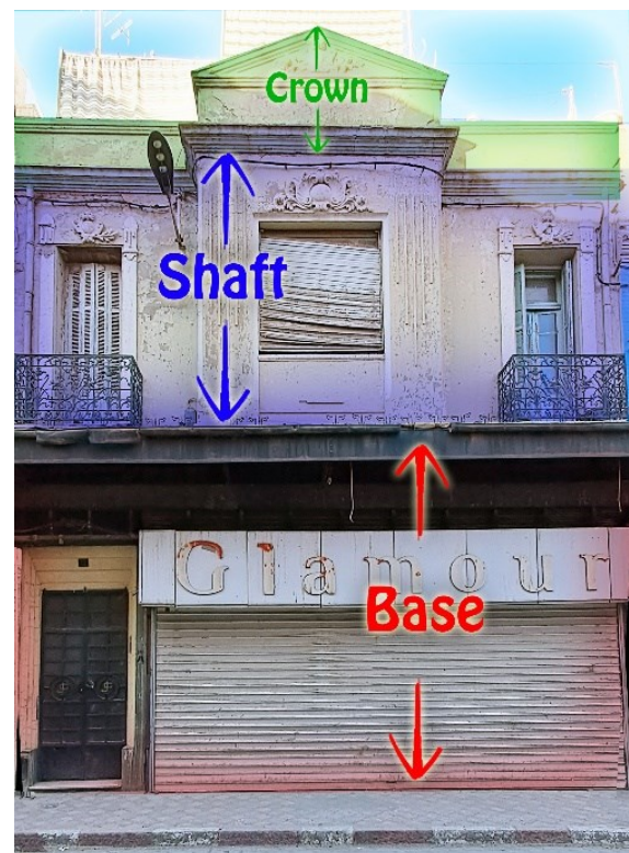
Fig. 3. Tlemcen's facade tripartite composition, which is a classical architectural concept that divides a building's facade into three distinct horizontal sections. It was used in the Tlemcen colonial facades to create balanced and aesthetically pleasing designs. (Source: Authors, 2024)
