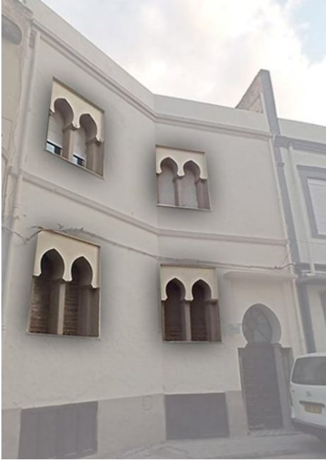
Fig. 21. Examples of geminated windows in Tlemcen. They are pairs of windows that are closely set together, sharing a central column or a mullion. This design element draws from traditional Moorish architecture, incorporating intricate and ornamental details. (Source: Authors, 2024)
