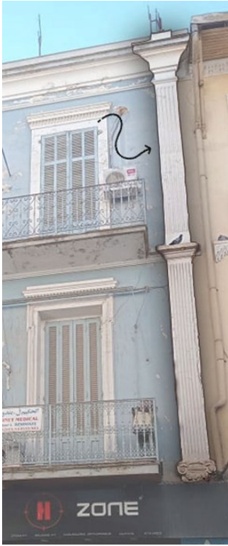
Fig. 4. A fluted pilaster with a Doric capital which is a vertical, rectangular element that projects slightly from the wall. The surface of the pilaster is adorned with vertical grooves, known as flutes, which add texture and visual appeal to the colonial facade. (Source: Authors, 2024)
