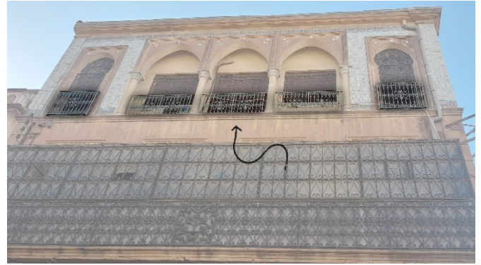
Fig. 19. An example of an insulated balcony in typology B. (Source: Authors, 2024)
