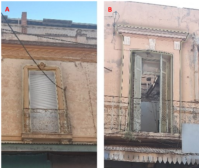
Fig. 8. Examples of French windows designed to provide abundant natural light and unobstructed views while adding an elegant and classic look to the space. They are commonly used to connect interior spaces with outdoor areas such as gardens, patios, or balconies. A) A central clasp in the moulded frame of a French window; B) A straight pediment above the French window. (Source: Authors, 2024)
