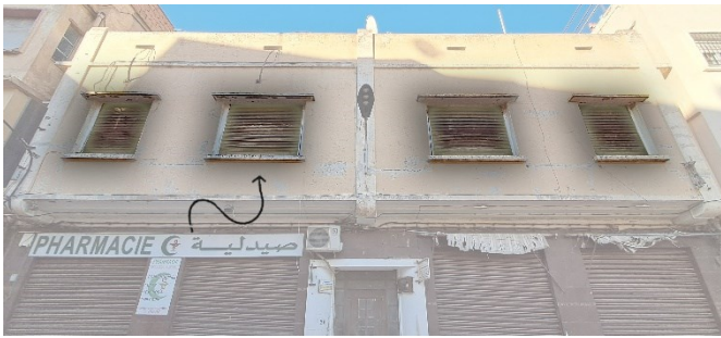
Fig. 24. C typology windows with sills and awnings. (Source: Authors, 2024)
