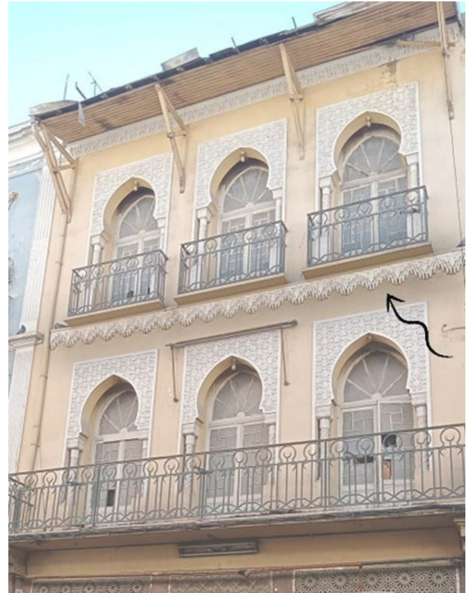
Fig. 20. A horizontal line of Muqarnas. Muqarnas consists of intricate, repeating geometric shapes that create a three-dimensional, tessellated pattern. When arranged in a horizontal line, these shapes form a continuous band of decorative elements that can vary in depth and complexity. (Source: Authors, 2024)
