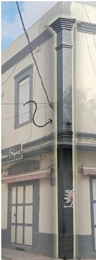
Fig. 5. An example of a corner chain which consists of a series of vertically aligned stones that mimic the appearance of a chain. Corner chains in colonial facades are often used to add visual appeal and emphasize the edges of a building, creating a sense of strength and stability. (Source: Authors, 2024)
