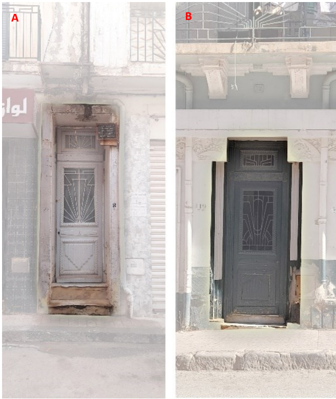
Fig. 10. Sub-type 2 types of doors are characterized by their bold geometric patterns, often found in the panels or glass inserts. The most popular decorative element is often radiating from the central point of the door. (A, B) Wooden doors with geometric iron detailing. (Source: Authors, 2024)
