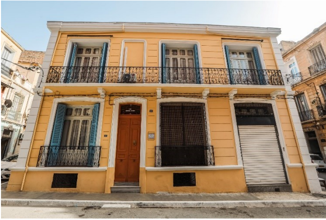
Fig. 3. The façade of the house after restoration. (Source: Sifeddine Kaddouri, 2022)
