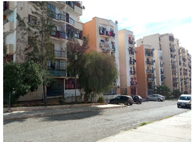
Fig. 3. View of the rear façade. (Source: Authors, 2023)
