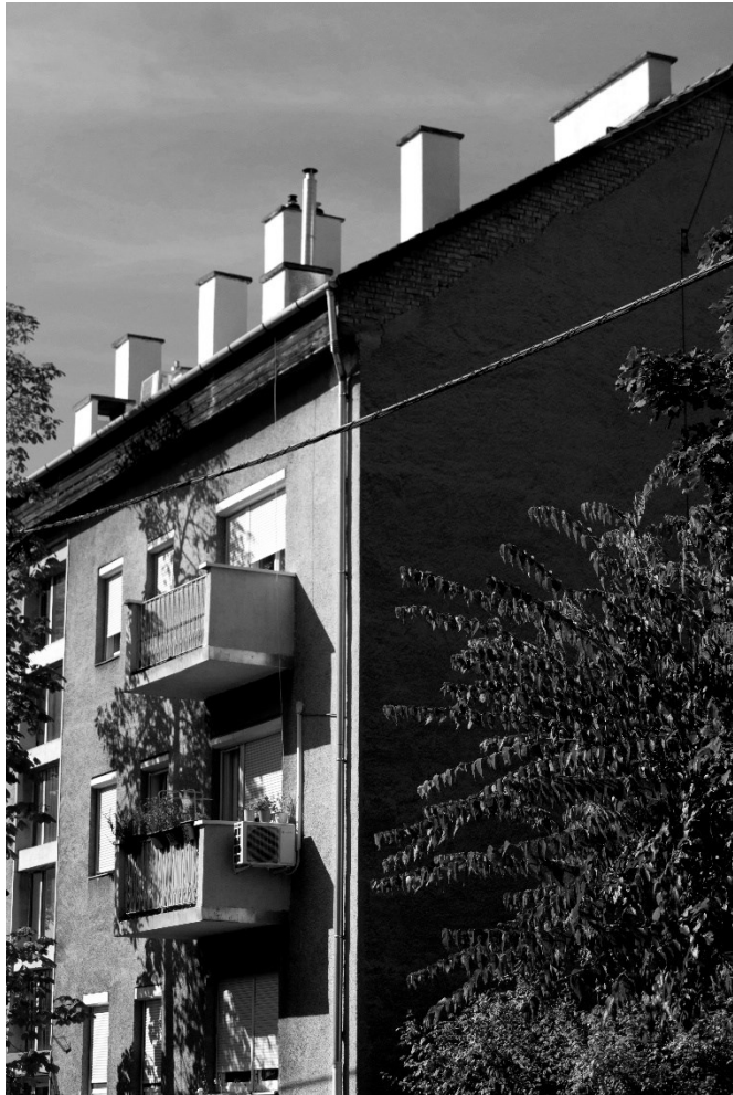
Fig. 18. Façade detail of the Adria Street small HE. (Photo: Author, 2023)
