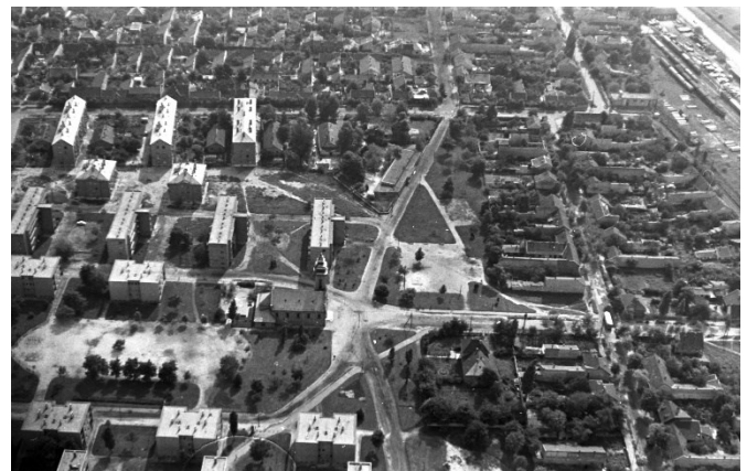
Fig. 4. Aerial view of the Béke Square small HE in 1963. (Photo: MHSZ, 1963)
