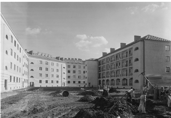
Fig. 10. The Hunor - Vihar Street small HE during its construction. (Photo: UVATERV, 1956)
