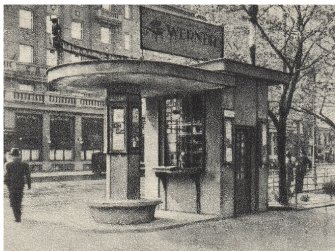
Fig. 7. Rudolf Frič, Tram shelter with kiosk of Kazimír Polák, Hviezdoslavovo Square, Bratislava, 1928. (Photo: Frič's personal possession, author's personal archive)
