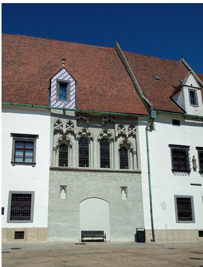
Fig. 11. The middle part with the reconstruction of medieval surface. (Photo: Author, 2023)
