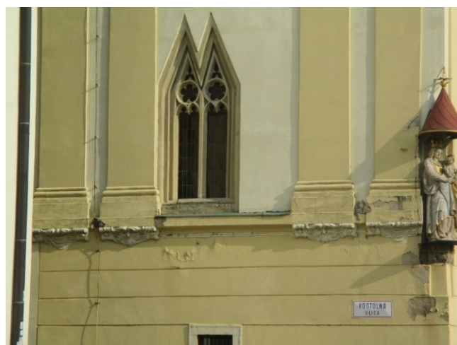
Fig. 18. Detail of rich plastic bifora with wimperg on the first floor. (Photo: Author, 2020)
