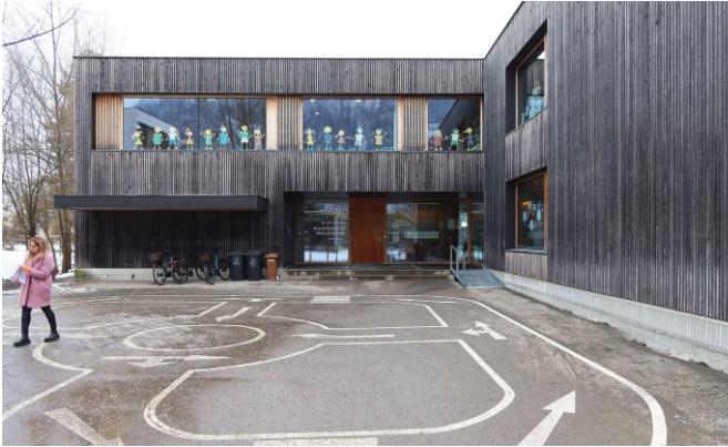
Fig. 10. The photograph shows a recess with entrance. On the facade, one can see how the wood authentically changes when directly or indirectly exposed to weather conditions. (Photo: Jakub Hanták, 2023)
