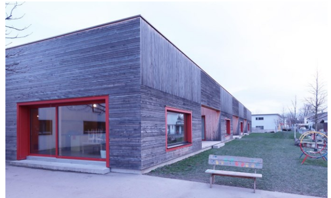
Fig. 2. A view of a ventilated facade that has naturally changed to a grey shade due to weather exposure. (Photo: Jakub Hanták, 2023)
