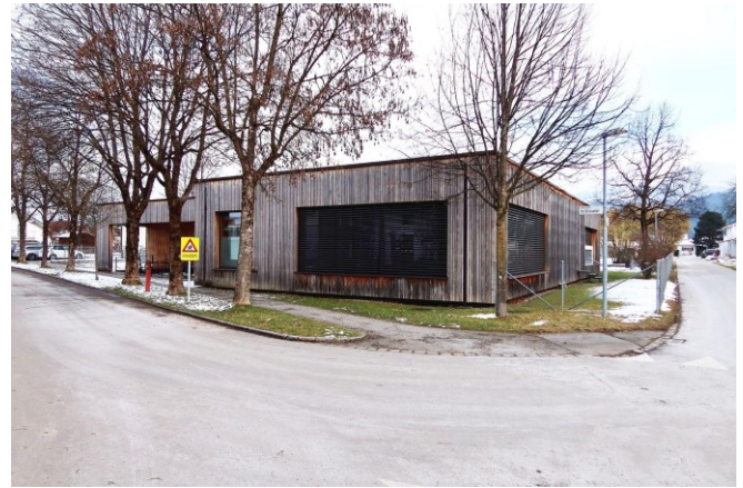
Fig. 14. The extension of the kindergarten building with a wooden cladding in Im Grisseler Street in the city of Feldkirch. (Photo: Jakub Hanták, 2023)
