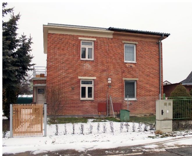
Fig. 11. House type Šimonovany. The left side has been reconstructed with regard to the values of Baťa architecture. The right side has been reconstructed regardless of the values of the Baťa architecture; it is obvious the original windows have been replaced. (Photo: Veronika Vaňová, 2022)
