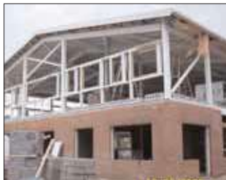
Fig. 48: Chaul End Centre – external brickwork construction.
