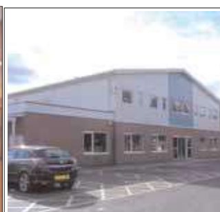
Fig. 51: Chaul End Centre – completed external works.
