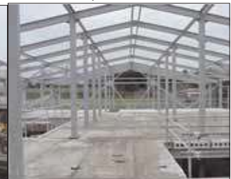
Fig. 47: Chaul End Centre – erection of pre-cast floor units.
