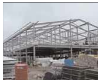
Fig. 46: Chaul End Centre – erection of steel frame.
