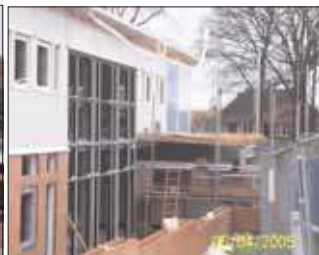
Fig. 49: Chaul End Centre – installation of cladding, curtain walling and windows.
