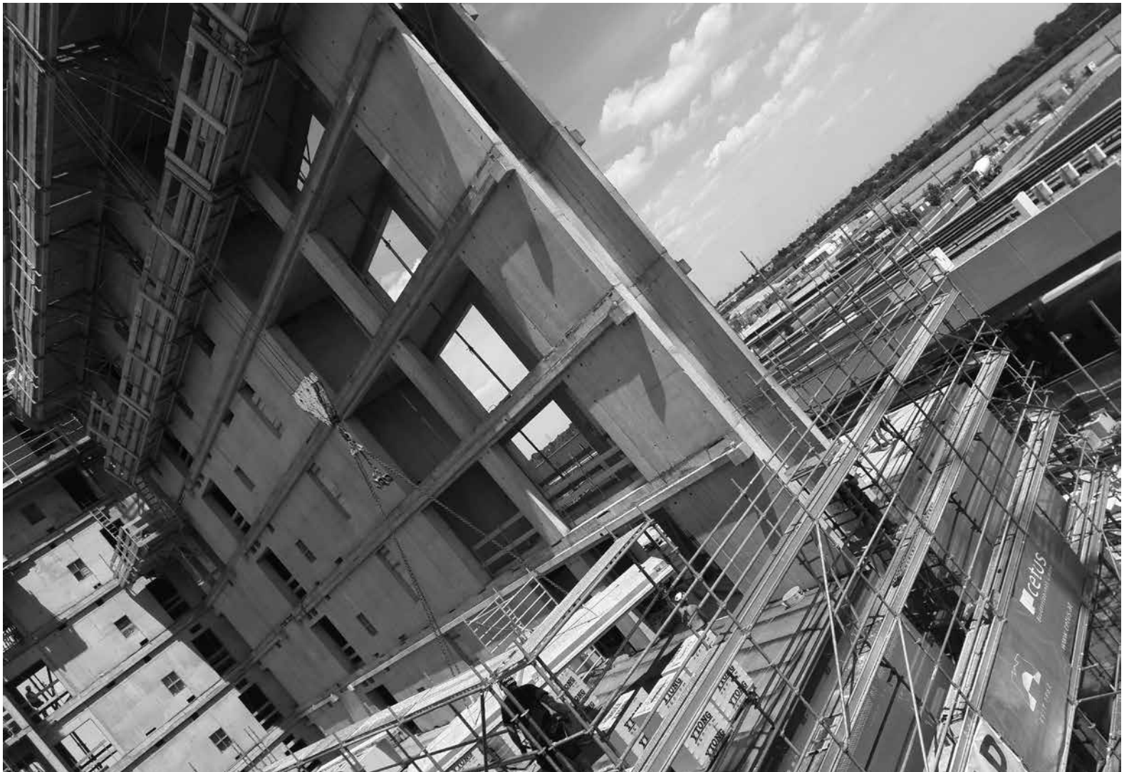
6 HoHo Vienna, the concrete core
